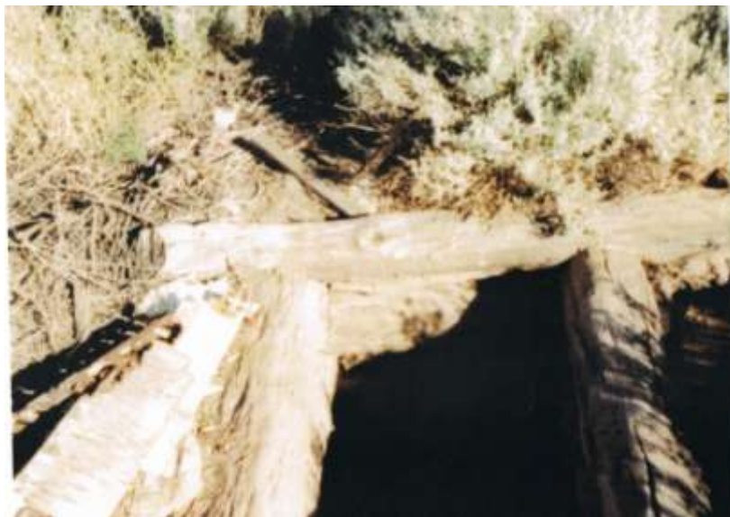
Figure 7: A native well shored up and rehabilitated by National Mapping (ICSM)
